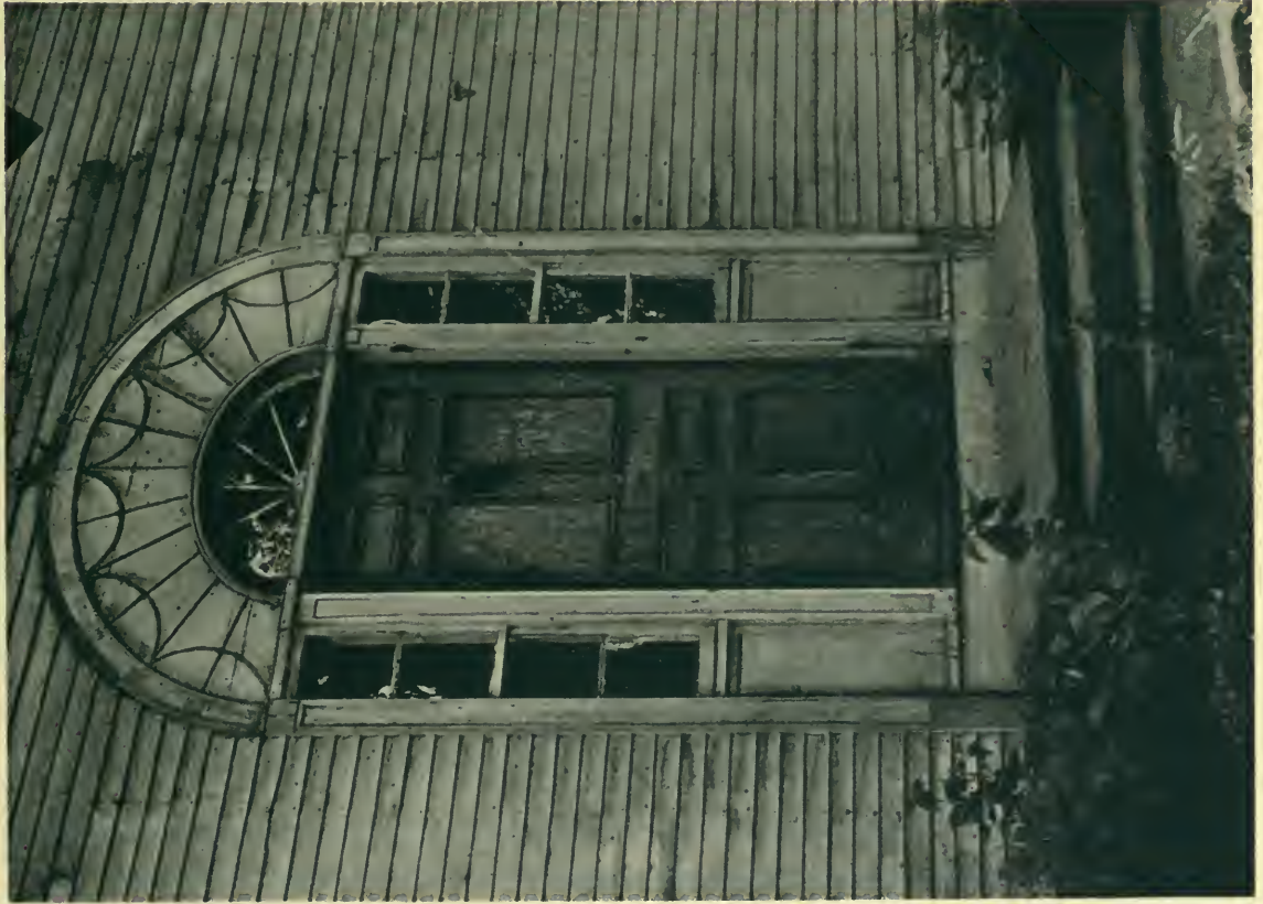
FRONT DOOR DETAIL, THE SMITH HOUSE, DEERFIELD, MASSACHUSETTS.
